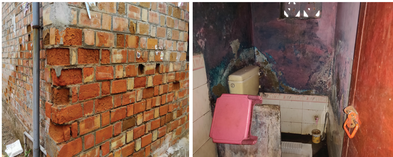
Figure 6: Cracks on the external walls of the buildings indicating poor quality of construction and Poor maintenance of drainage system and common areas
