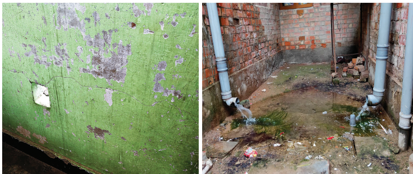
Figure 6: Cracks on the external walls of the buildings indicating poor quality of construction and Poor maintenance of drainage system and common areas
